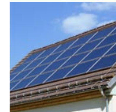
Premium in-roof construction with 28 modules and a total output of 9 kWp
