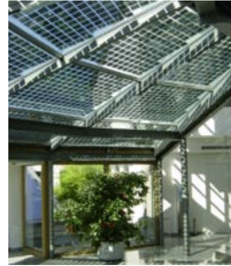
Aluminium skylight construction – internal view. 147 m 2 module surface
