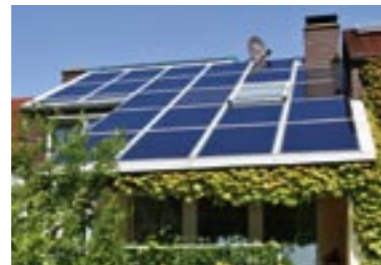
Premium complete roof construction, 22 modules and integration of a roof window
