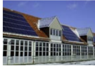
PV-Light on-roof construction with 120 modules
