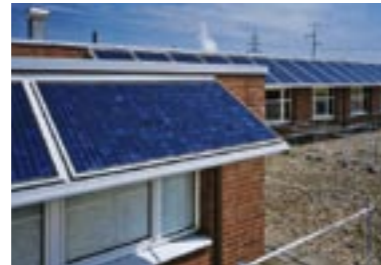
Premium canopy construction with a total output of 7 kWp
