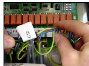
12. Connect the sensor cables of tanks 1 and 2 to the filling level electrodes (luster terminals) (view from front):
